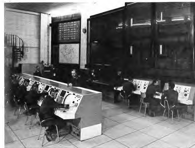
NATO Bunker—This main operations room of a NATO bunker on the Belgian-Netherlands frontier is one of four custom-tailored air defense "nerve centers" to be installed in the countries of Belgium, West Germany and The Netherlands to provide each nation with integrated, split-second, computerized protection against aerial attack.
