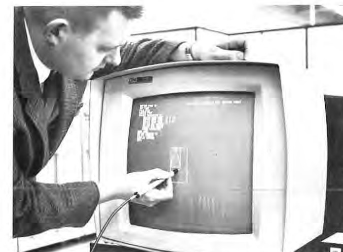
Operator has just defined a character on an IBM 2250 Display Unit, using a font-design program. The nine primary commands and one set of secondary commands used to direct program are displayed in upper left-hand corner of screen.
