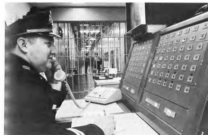
Captain Kirkwood S. Wyatt, correctional officer at Baltimore City Jail, makes administrative call while scanning Security Alarm System console for reporting calls. Signal lights at bottom of consoles indicate purposes of calls made from security phones. Miniature displays represent phones throughout the facility.
