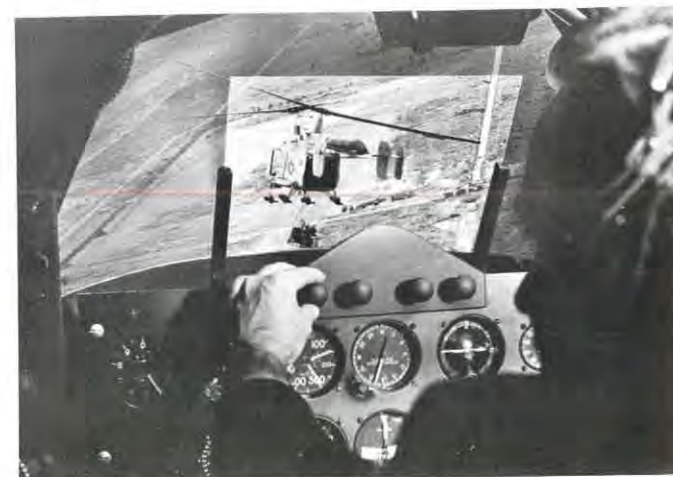
Simulated installation of "Night Window" showing pilot getting clear view of helicopter landing on twilight-shrouded field.
