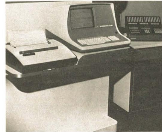
The Energy Communications Service printer provides periodic and demand reports of energy load status (left); the Energy Communications Console is the control center from which energy usage can be modified (center); the Dimension PBX console is used to control the communications for the facility (right).
