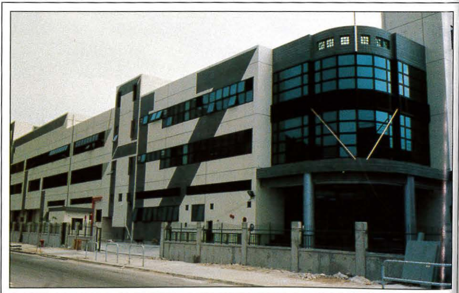
Fig. 1: Varitronix moved into its new 160,000-ft. 2 manufacturing facility and headquarters in Hong Kong's Tseung Kwan O Industrial Estate in October 1997.
