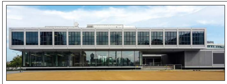
Fig. 5: The facade of the Merck KGaA/EMD Innovation Center in Darmstadt, Germany, uses switchable licrivision smart windows. Photo: Merck KGaA
