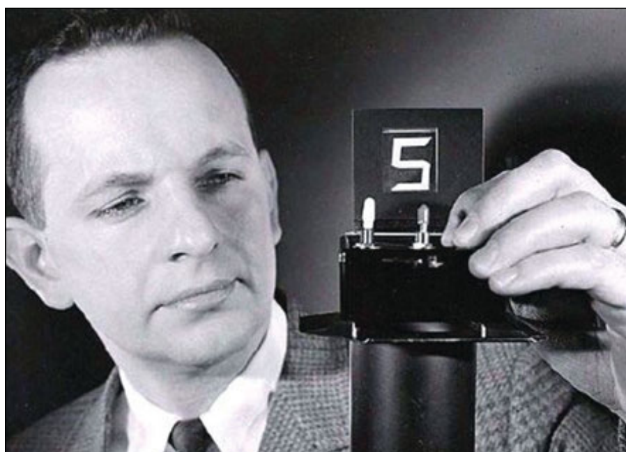
Fig. 1: This early LCD (with inventor George Heilmeyer) may look primitive, but it was a revelation back in the 1960s.
